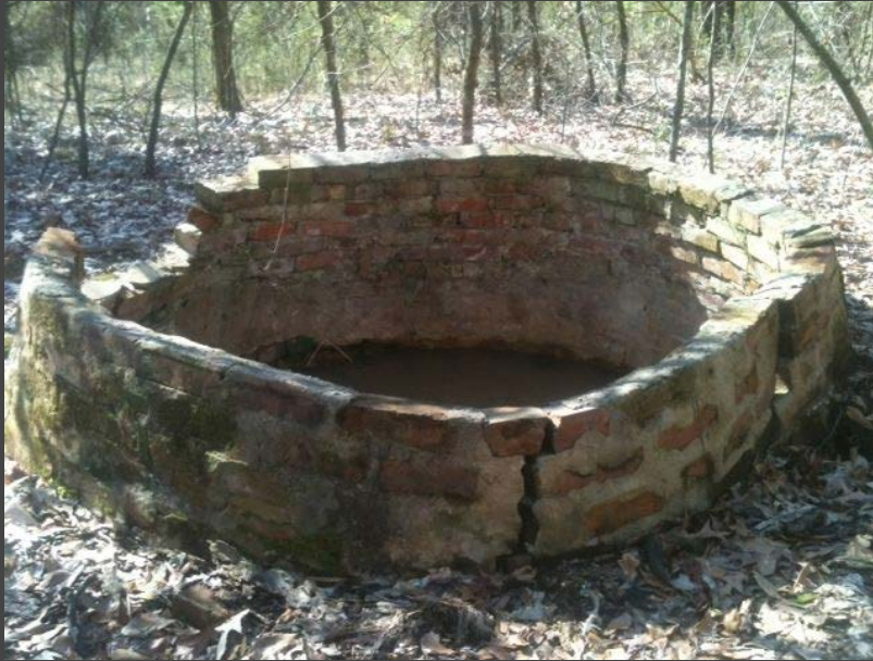
Cistern near Natchez Trace, Mississippi
